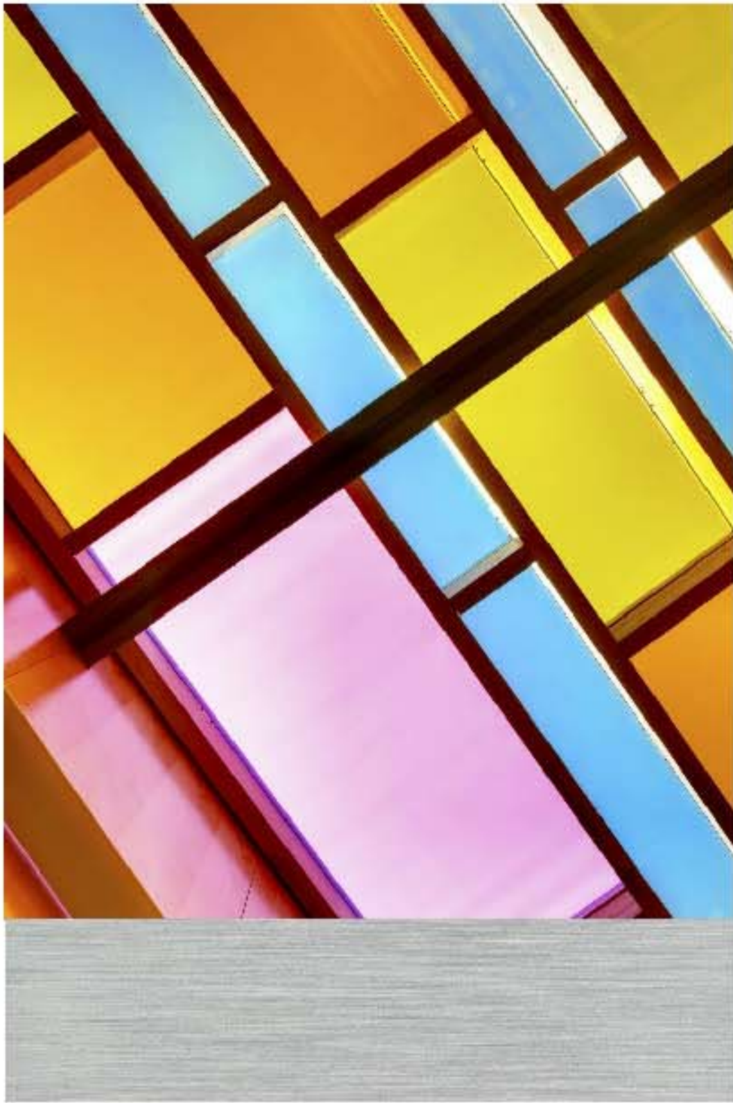
Feature Glazing Coloured glazing film to Low-E double glazing
