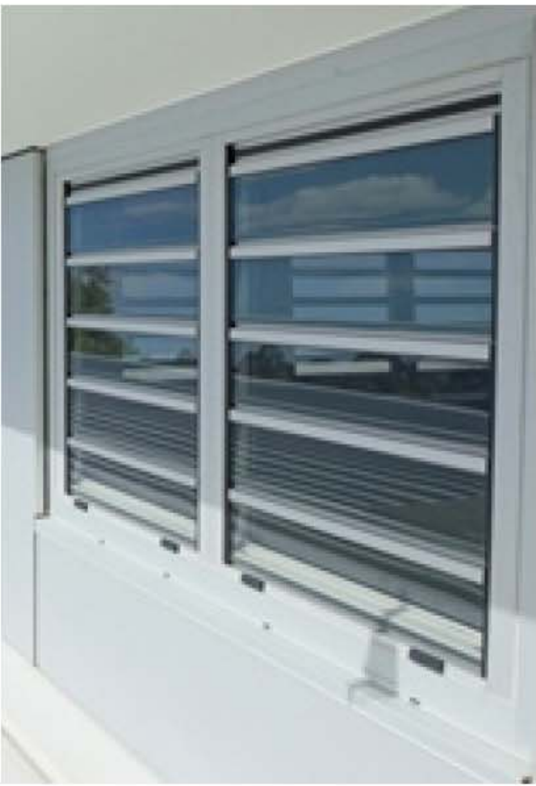
Anodised aluminium frame louvre windows to homebases
